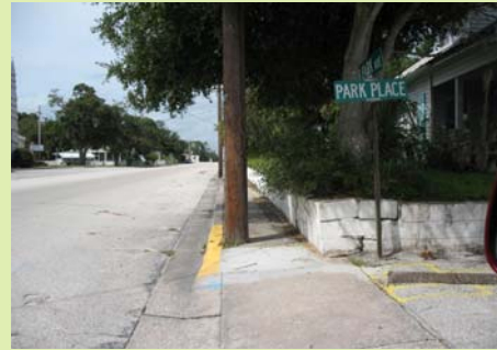
Some sections of the sidewalk along Park Avenue do not provide clearance for users
