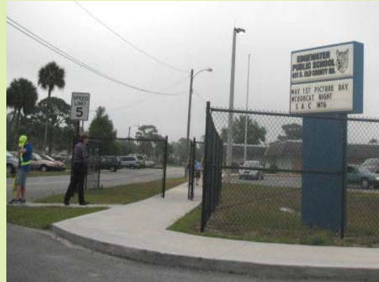
The new sidewalk on campus needs a curb ramp
